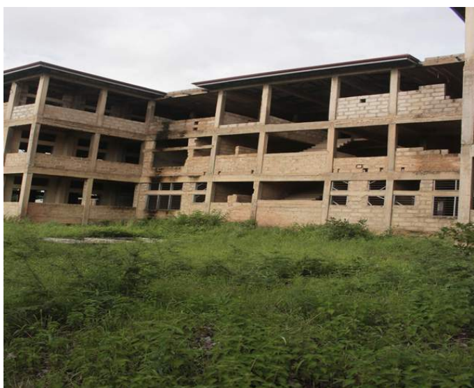
COURT COMPLEX UNDER CONSTRUCTION.
